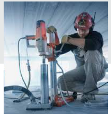
Concrete Core Extraction
