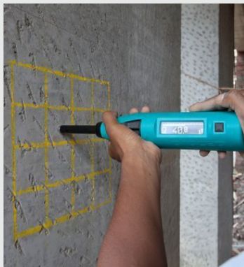
Rebound Hammer Test
